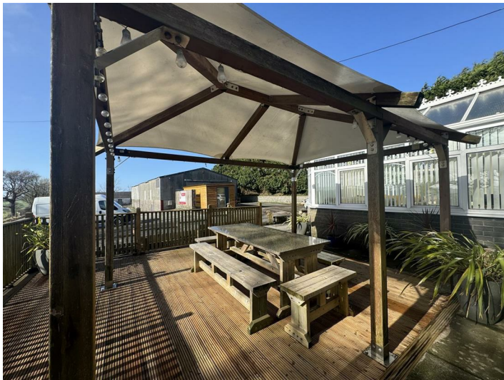
Driveway and vehicular hard standing areas leading to garage. Covered decking to the fore together with front and side garden predominantly laid to lawn.
